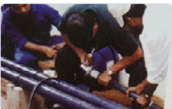
Cleaning residential heating pipes
