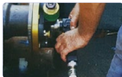
Cleaning pipes and tubes
