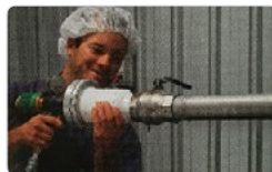
Cleaning pipes of various manufacturing and industrial facilities
